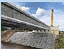
RC Post / Prestressed Tensioned Girders
