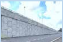
Reinforced Earth Wall
